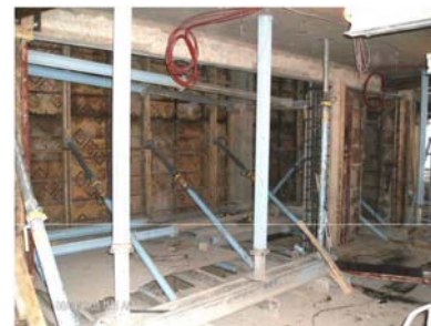
Shear wall formwork and bracing
