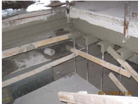
Fire proofed structural steel around stair opening
