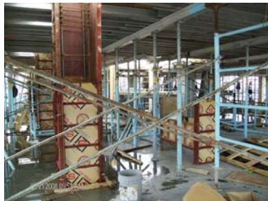
Column formwork
